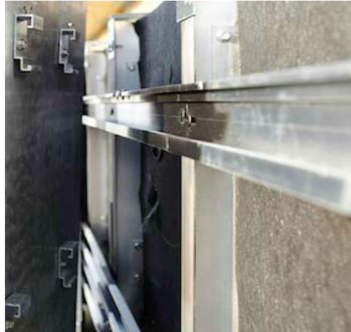
Mounting the tile onto the supporting construction Photo: KEIL Befestigungstechnik
