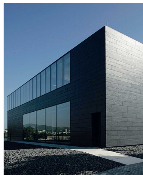
Rathscheck office and training building, Mayen, DE © Rathscheck Schiefer
